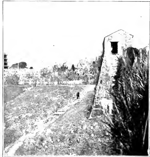
Old Wall, Canton (now demolished)
